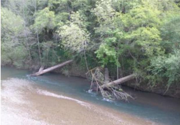
**Stream flow around these installed large wood, root wad, and boulder structures scours gravel out downstream of the structures to form deep pools and cover for adult and juvenile salmon.**
